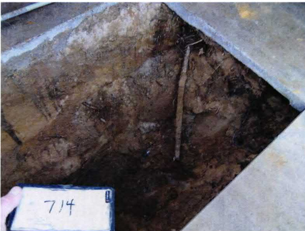
Picture 2: UST 714Bluebell excavation.
